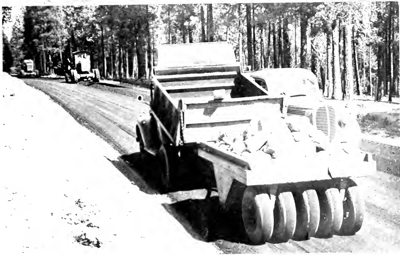
At top—Easy going on 40,000 lb. log load. Bottom—Spreading gravel for dirt surface with grader for road bed.
